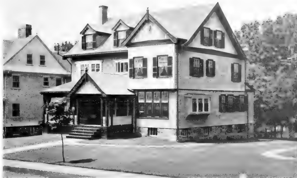
1—A House of Good Style with Shingled Sides, and Half-Timbered Gable Ends
